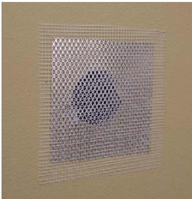
For larger holes or indentions (golf ball sized or larger), use a metal drywall patch kit to reinforce the hole (sold at most hardware stores). Spread a thin layer of drywall spackle over the surrounding area, place the reinforcing patch on the area to be repaired, and then apply a few thin coats of spackle over top of the patch, allowing each to dry completely before adding more spackling. When dry, sand the surface with fine grain sandpaper before painting.
